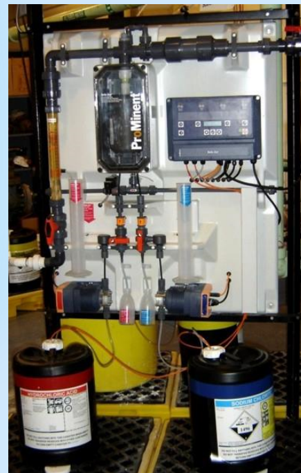
Chlorine dioxide generator in Holland, MB
